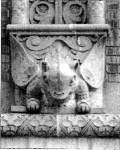
One of a pair of terra cotta squirrels above each of the 4th floor projections.
